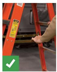
Properly set-up and use the ladder in accordance with safety instructions and warnings. Wear shoes with non-slip soles. Center body on the ladder and keep belt buckle between the rails while maintaining a firm grip. OSHA has a Quick Card available on ladder safety. This could be a topic for a tailgate safety meeting. <a href="https://www.osha.gov/sites/default/files/publications/portable-ladder-gc.pdf">https://www.osha.gov/sites/default/files/publications/portable-ladder-gc.pdf</a>
